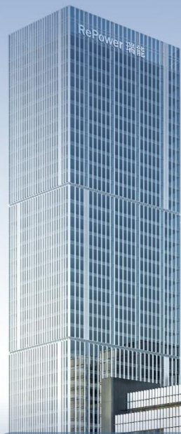
Repower Headquarters, R&D and Customer Service Center
